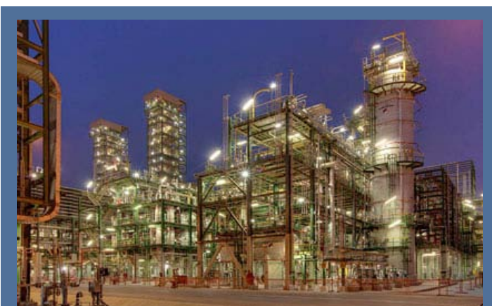
Linde-Polyethylenanlage in Jubail/ Linde Polyethylene-Plant in Jubail
