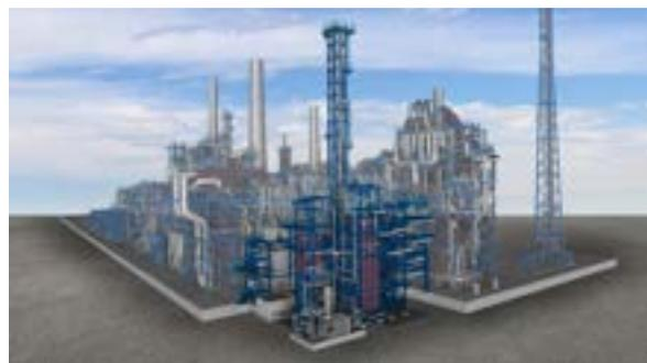
It features two distinct demonstration furnaces exploring different heating methods: direct heating, which allows electric currents to flow through cracking coils, and indirect heating, which uses radiative heat from surrounding elements. Together, these methods process approximately 4 tons of hydrocarbon feedstock per hour, underscoring the plant's substantial contribution to decarbonization.
