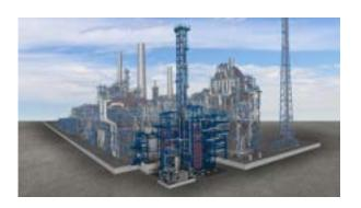
It features two distinct demonstration furnaces exploring different heating methods: direct heating, which allows electric currents to flow through cracking coils, and indirect heating, which uses radiative heat from surrounding elements. Together, these methods process approximately 4 tons of hydrocarbon feedstock per hour, underscoring the plant's substantial contribution to decarbonization.
